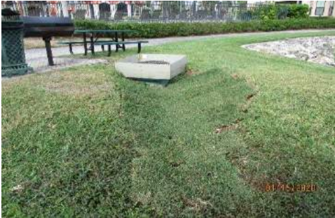
New Grading around Catch Basin
