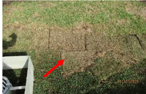
Sod Dying around Catch Basin
